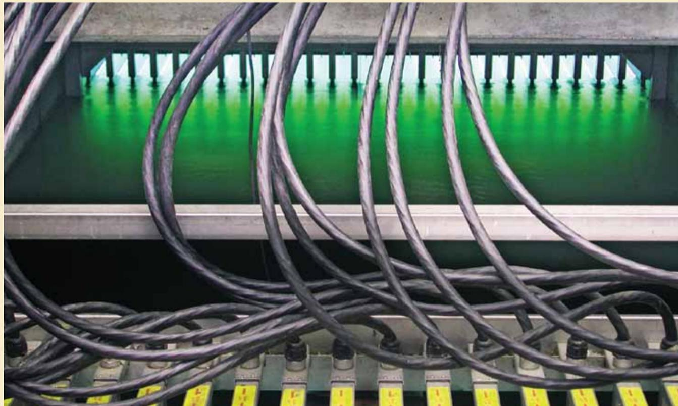
Wastewater is disinfected when it flows past submerged UV lamps.
