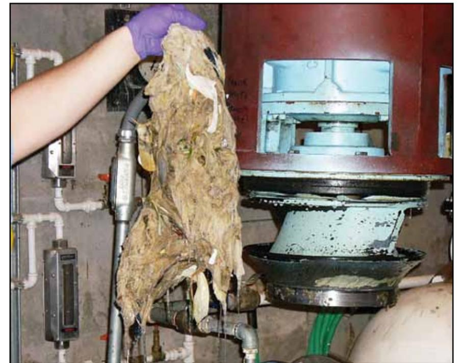
Nasty clumps of so-called disposable wipes—like this one that was clogging up our equipment at the Moraga pumping station—are requiring us to spend more time and money on maintenance and repair work.
