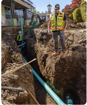
Replacing your lateral using polyvinyl chloride (PVC) pipe or pipebursting can reduce the risk of root intrusion, cracks, joint misalignment, and general leakage.
