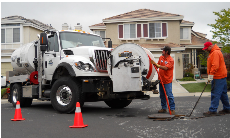
Collection System Crew Cleaning a Sewer
