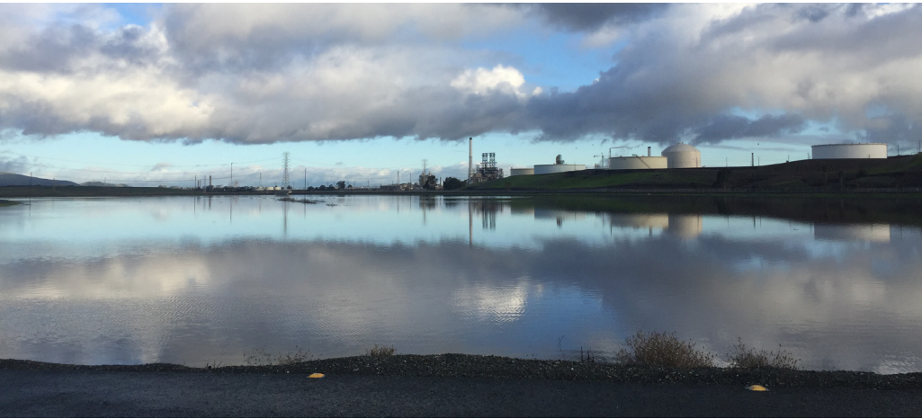
Wet Weather Holding Basin B During a Recent Storm Event
