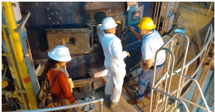
Inspection of the Multiple Hearth Furnaces
