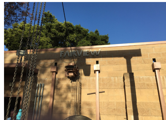
Fairview Pump Station
