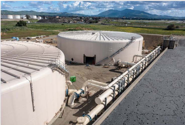
Constructing new steel storage tanks and replacing electrical gear under the Filter Plant and Clearwell Improvements – Phase 1 Project
