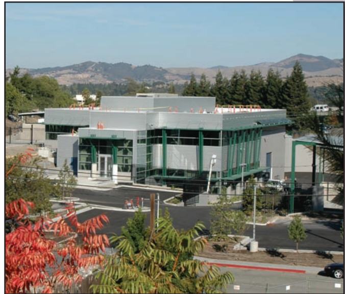
Our new facility in Walnut Creek is nearly completed.
