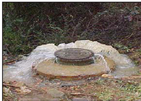
This is an actual sanitary sewer overflow caused by an oil and grease blockage.
