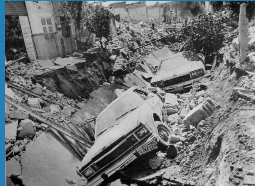
1992 – Guadalajara, Mexico. More than 250 fatalities, 5 miles of city streets destroyed – sewer explosions resulting from flammable liquid (gasoline) discharge
