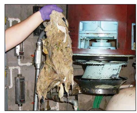
Nasty clumps of so-called disposable wipes—like this one that was clogging up our equipment at the Moraga pumping station—are requiring us to spend more time and money on maintenance and repair work.
