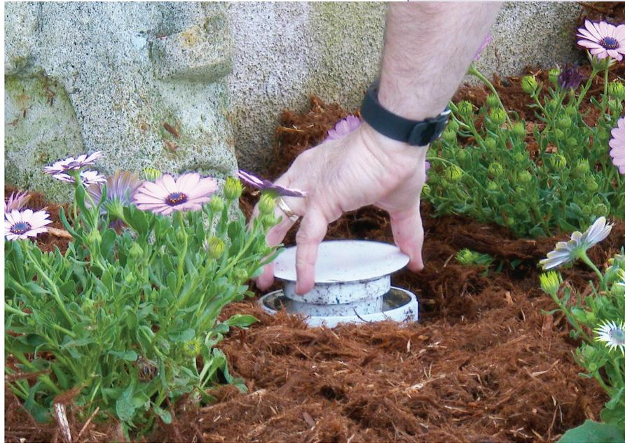
Overflow Protection Devices are available at plumbing supply stores. We recommend installation by a licensed plumber.
